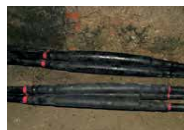
24CSJ cold-shrinkable straight joint
