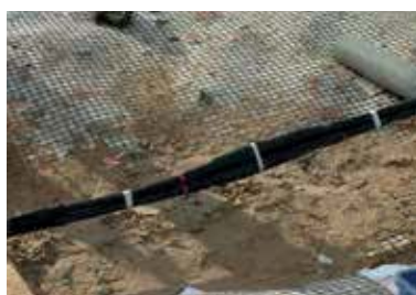
TS-24CSJ hybrid transition joint
