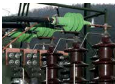
AFN10 as a transformer connection
