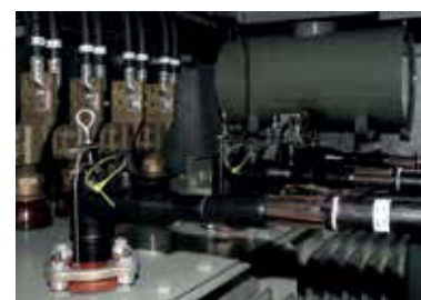
Transformer connection with 158LR
