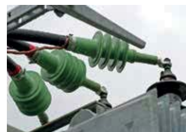
AFN20 as a transformer connection
