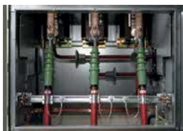
AIN20 with compression cable lug
