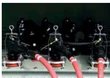
Transformer connection with 158LR
