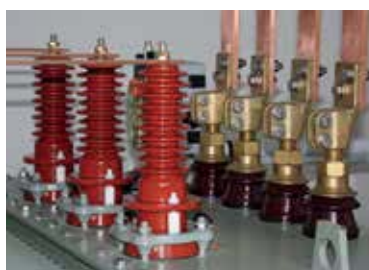
PITO-E on transformer with bushings
